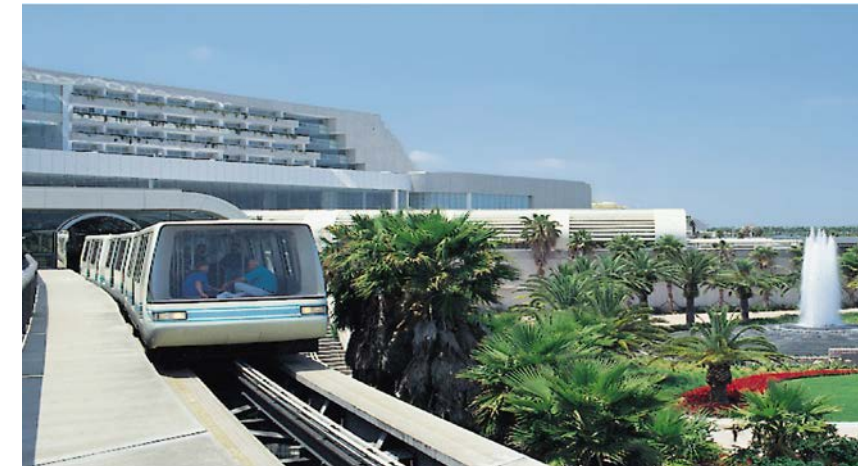
Automated People Mover (APM)
